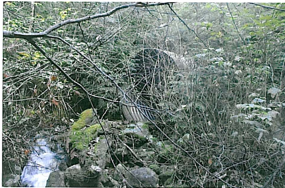
CK-2349 Outlet Overflow Pipe
